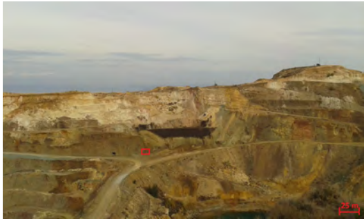
Figure 8: The Phoukasa main ore deposit to the right, the Skouriotissa fault lies roughly parallel along the NW going road, and the Phoenix deposit lies to the left. The dark brown/black sedimentary layer is the sulphide lying on top of the stockwork. The red box indicates sampled area for DTC151205. Photo is taken towards the north. (Photo Diana Carlsson)
