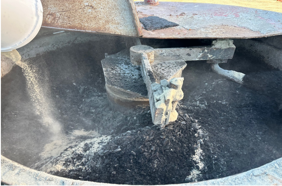
Fig. 18 A picture of the mixer with the dry materials, already added is the biocarbon, mill scales, chromite ore, cement, and dust, the binders are being added while mixing is taking place.
